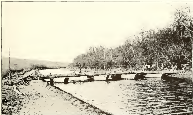
THE HEAVY PONTOON BRIDGE ACROSS THE MEUSE CANAL AT BRIEULLES. ONE OF THOSE CONSTRUCTED BY FRED D. MENDENHALL, '14
